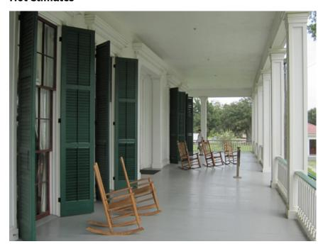
For buildings in hot climates that do not require any additional heating, extend shading devices to cover the entire south façade and adjacent occupied outdoor areas. This creates and allows for indooroutdoor spaces and the use of sheltered outdoor areas yearround.
